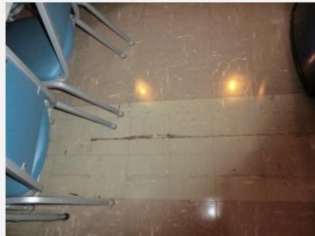
Separation in floor slab / cracked asbestos flooring
