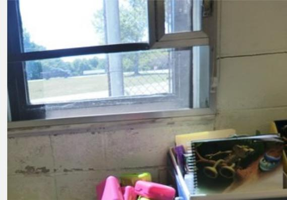
Crack and moisture damage in classroom walls
