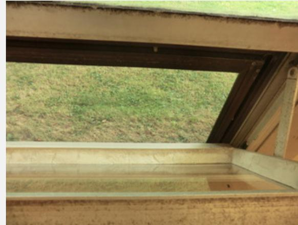
Single pane windows have deteriorating seals and fail to close properly
