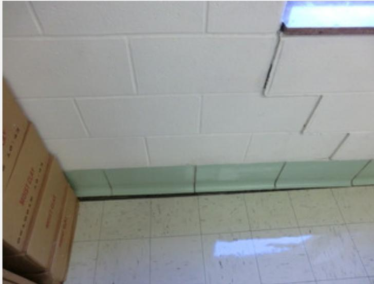
Wall cracking & separation between floor & wall
