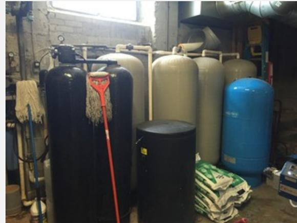
Well water system cannot support a fire sprinkler system
